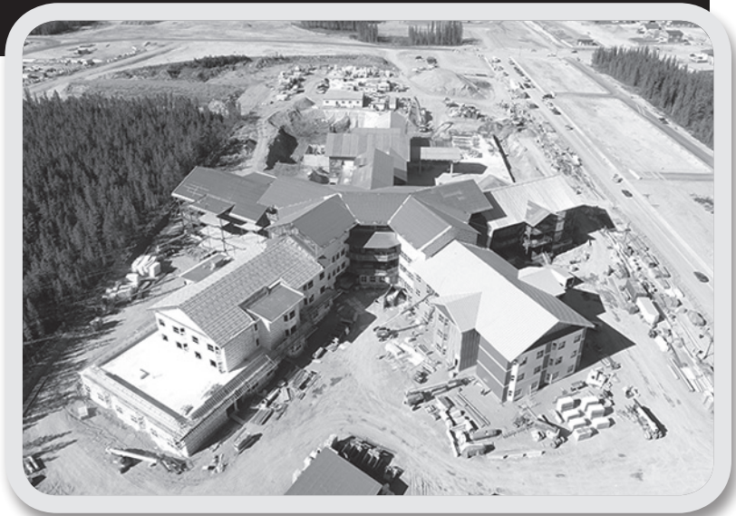
▲ Whistle Bend Continuing Care Facility Drone Photo: August 9, 2017
